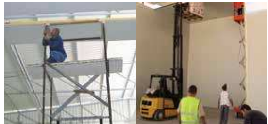
The mounting of the cold storage is complete when the ceiling has been mounted.
