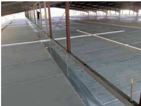
Ceiling sponder and joints used to connect the ceiling panels
