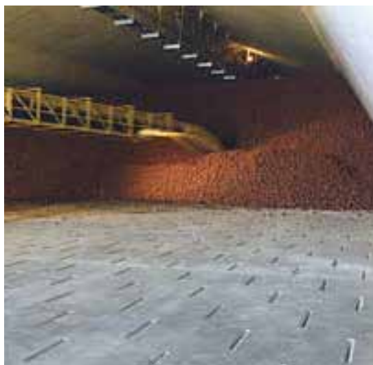
Air canals for storing onions in bulks
